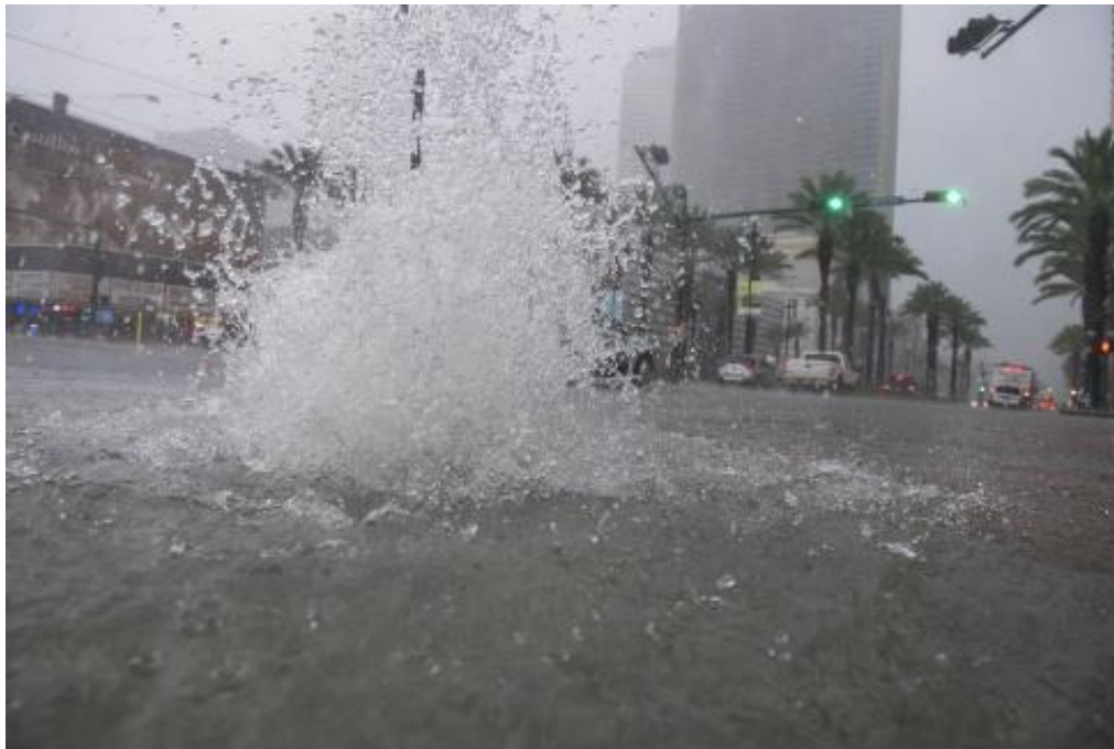
Photo 14 Manhole overflowing at Canal-Tchoupitoulas intersection: 14. Manhole
