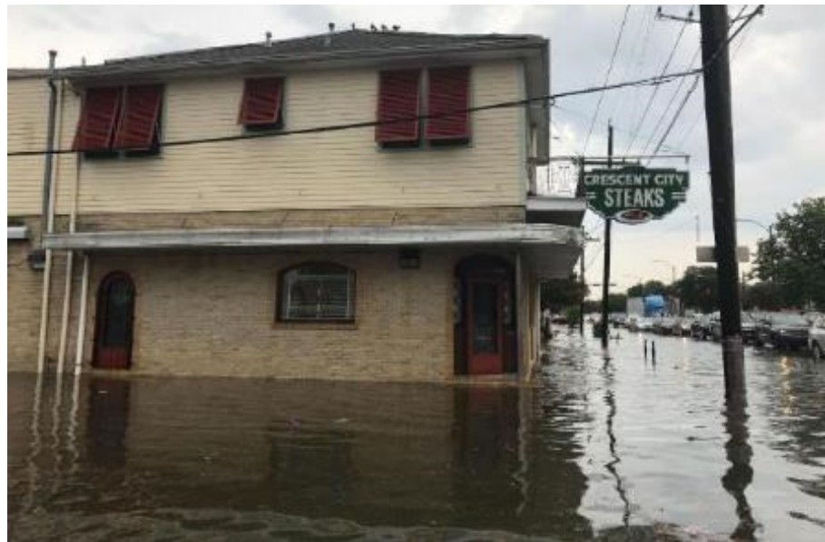
Photo 8 Flooding outside business in Treme/LaFitte (1001 N. Broad St.): 8. Crescent City Steaks
