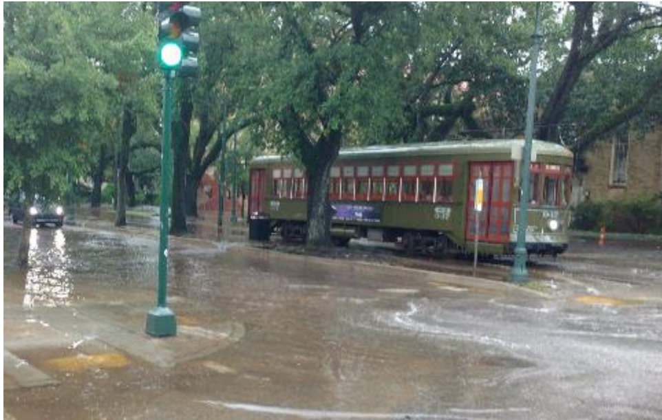
Photo 1 Street Flooding on St. Charles Ave.: 1. St. Charles near Broadway
